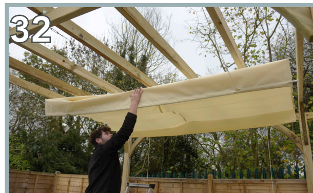
32 The Large and Small Ropes tied to the Pole will look like the above. Once both ropes are tied to the pole, push the whole Canvas towards the back of the Pergola.
