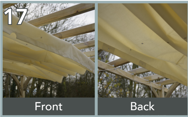
The front of the Canvas has 2 x rounded cutouts and the back has eyelets for screwing into the rafter. For reference, see the above.
