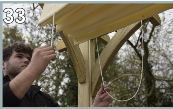
33 Ensure the Long & Small Ropes on the back of the pergola, are pulled over the top of the Canvas as shown above.
