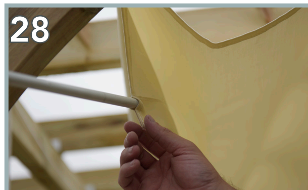
28 Using the other Pole Section, insert it into the small hole on the opposite edge of the Canvas, as shown above.
