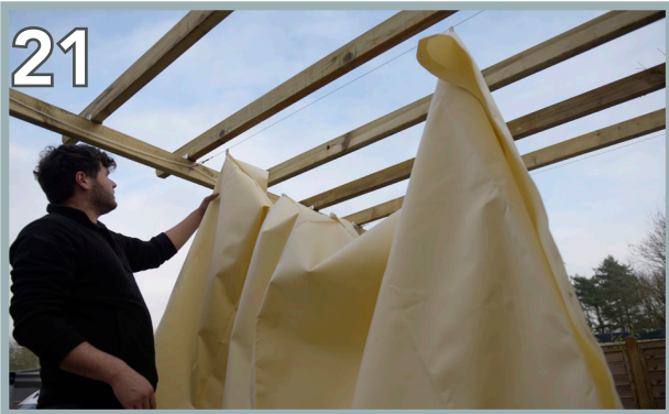
Fold out the Canvas and hook the remaining clips along the middle Wire.
