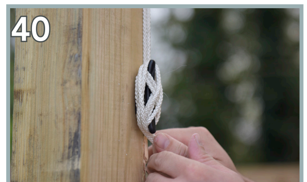
40 When opening or closing the pergola, make sure to tie up both tied Ropes to the Plastic Cleats, as this will ensure the Canvas is always taught. Ensure any trailing rope is secured to the fixings provided.
