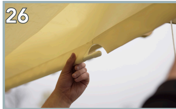
26 Once inserted, slide the Pole Section back to the sealed edge of the Canvas.
