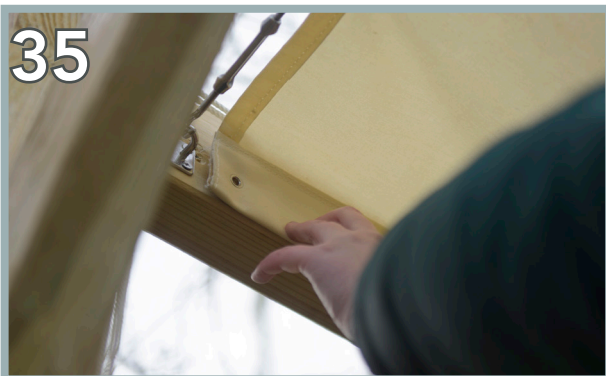
35 Position the back of the Canvas onto the back rafter. Ensure the Canvas is taught along the edge.
