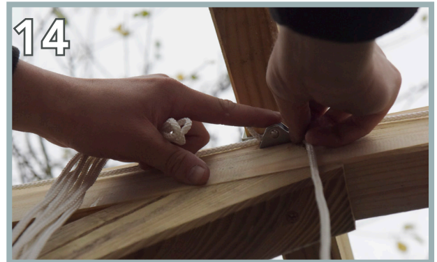
Using the 1 x Small Rope, thread one end through the Small Roller closest to the Large Roller on the front of the pergola. Repeat this on the back.
