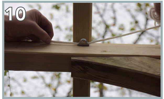
Once secured, take 1 x Long Rope and thread one end through the Small Roller furthest away from Large Roller. If necessary use a finger to feed the rope through the Roller.
