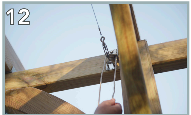
Thread the Long Rope through the top of the Large Roller and pull it through the bottom. Ensure the other end of the rope does not leave the Small Roller.
