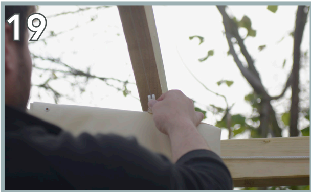
Take the plastic clips from the middle of the Canvas and start from the back. Place the clip around the middle Wire and twist it to hook it on.
