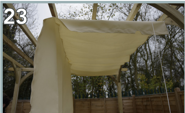
Repeat the process for all of the remaining plastic clips on both edges of the Canvas, as show above.
