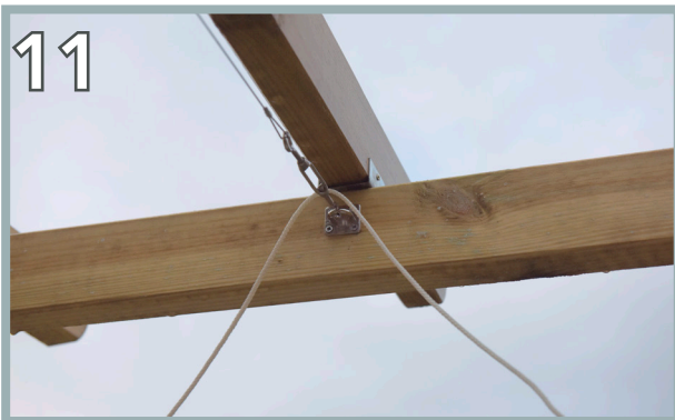
Ensure the Long Rope goes over the top of the middle Wire, as shown above.
