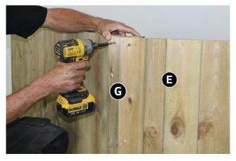
Fix Roof Capping (G) to Roof Panels (E) using 4x 35mm screws (2x 35mm at each end)
