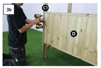
Position 1x Back Panel (D) in to base of block stopper in side panels and fix using 4x 40mm screws (2x screws per side).
