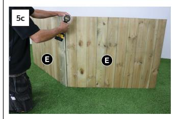
Attach remaining Roof Panel (E) using 2x 60mm screws as shown in Fig. 5c (1x 60mm screw at each end).
