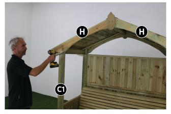
Locate roof assembly onto Side P anel (C1 & C2) posts and fix in position using 8x 50mm screws (2x 50mm screws per post).
