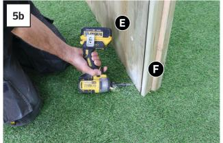
Attach 1x Roof Panel (E) to Roof Support (F) using 2x 60mm screws as shown in Figs. 5a & 5b. **Note: Ensure roof board overlap are in correct orientation as to avoid rainwater ingress.**
