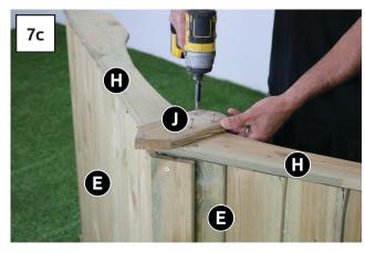
Set out 2x Fascia (H) as shown and attach to roof assembly using 6x50mm screws (3x50mm screws per fascia).
