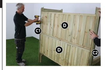
Position remaining Back Panel (D) as shown in Fig. 4 and attach using  $4x\ 40mm\ screws\ (2x\ 40mm\ screws\ per\ side)$
