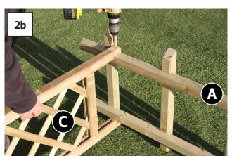
Locate Post/Trellis Assembly C onto Rails A as shown in Fig.2a (adjust width to suit). Fix in position using 2no 60mm Screws – 1no per side (Fig.2b).
