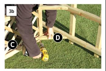
Ensuring Post/Trellis Assembly C is perpendicular to Rails A, position Bracings D as shown in Figs.3a & 3b and fix using 4no 50mm Screws – 2no per bracing.
