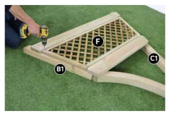
Set out Lower Leg (front) (B1), Upper Leg (front) (E1) and Leg (back) (C1) as shown (left) (large holes face down) and place Horizontal Long Brace (A) and Horizontal Short Brace (D) in position shown (Above left) Align bolt holes and insert 8 x 100mm Bolts. (Nuts & washers to be attached at a later stage).
