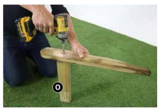
Align dowels in Armrest Support (O) with corresponding holes in Armrest (P1) and tap into position. Fix in place using 1x 60mm Screw.
