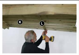
Insert Centre Batten (L) centrally beneath Canopy (K) and fix using 16 x 30mm Screws. (1 x Screw per slat), working from front to back.
