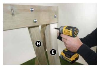
Ensuring Upper Legs (front) E1 & E2 are flush with underside of Swing Beam (G) (See above), fix to Legs (back) C1, C2 as shown using  $2 \times 100 \, \text{mm}$  Star Screws. (1 x Screw per leg).
