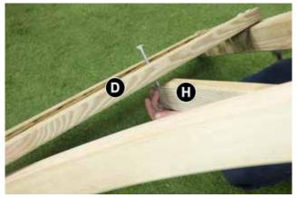
Attach Diagonal Brace (H) to Swing Beam (G) using  $2 \times 90$ mm Bolts, Nuts & Washers, and to Horizontal Short Brace (D) using  $1 \times 100$ mm Bolt, Nut & Washer.
