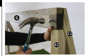
Attach other end of Swing Beam G to Back Leg C2 on previously assembled right hand side of swing using  $1 \times 100$ mm Bolt, Nut & Washer.
