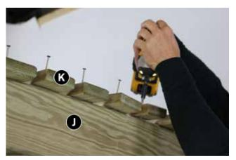
Set Canopy (K) out evenly on to Canopy Supports (J) and fix using 32 x 60mm Screws (2 x Screws per slat, 1x Screw at each end).
