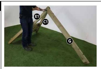
Ensuring large drilled holes are facing up, attach Swing Beam (G) to Back Leg (C1) using 1 x 100mm Bolt, Nut & Washer. Do not fully tighten at this stage.
