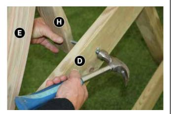
Attach remaining Diagonal Brace (H) to Swing Beam (G) using  $2 \times 90$ mm Bolts, Nuts & Washers, and to Horizontal Short Brace (D) using  $1 \times 100$ mm Bolt, Nut & Washer.
