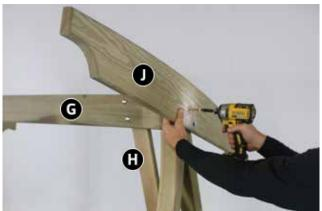
Attach Canopy Support (J) to Leg (back) (C1) using 1 x 100mm Bolt, Nut & Washer. Set at desired angle and fix to Swing Beam (G) using 1 x 80mm Screw.
