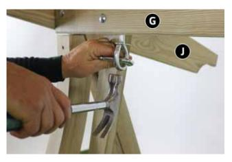
Insert 170mm Eye-Bolt into Swing Beam (G) as shown. Attach Washer & Nut and fully tighten. Repeat procedure with remaining 170mm Eye-Bolt on other side of swing.
