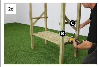
Attach 2x Side Frame Bracings (C) to Side Frames using 4x 35mm screws (2x per bracing), as shown in Fig 2. Ensure Side Frame Bracing (C) face outwards.
