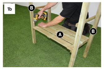
Fix Shelf Assembly (A) to Side Frames (B) as shown in Fig 1 using 4x 35mm screws. Ensure that shelf support rails face inwards.
