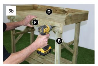
Attach Fascia Board (F) to Side Panels using 4x 35mm screws (2x per end), ensuring top of Fascia Board is flush with top of Worktop Assembly as shown in Fig 5a & 5b.
