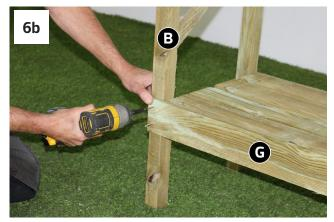
Position Shelf Upstand (G) to rear of Shelf Assembly and fix to rear legs of Side Frames using 4x 35mm screws (2x per end - See Fig 6).
