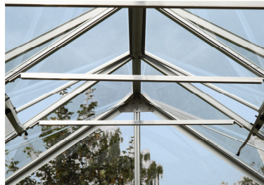
Strong braces at the roof and eaves
