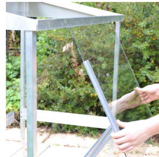
C. Fitting the glass
