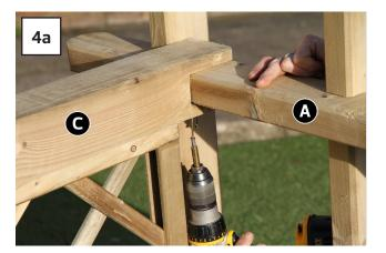
Position second Post C as shown in Fig.4 and fix to Rail A using 2no 70mm Screws. Fix Trellis Panel D to second Post C using 3no 60mm Screws.
