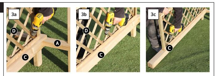
Place Trellis Panel D 90mm from top of Post C and fix in position using 3no 60mm Screws (Figs.3a,3b & 3c).
