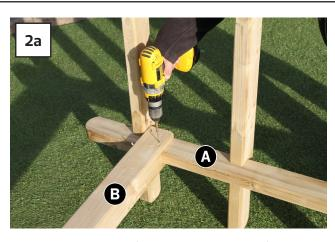
Locate Post C onto Rail A as shown in Fig.2a (adjust width to suit). Fix in position using 2no 70mm Screws.
