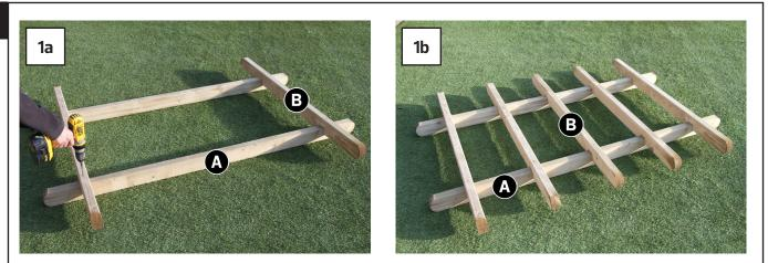
Position Rafters B 150mm from edge at both ends of Rails A and fix using 4no 70mm Screws – 2 per Rafter (Fig.1a). Space out remaining Rafters B evenly (Fig.1b) and attach using 6no 70mm Screws.
