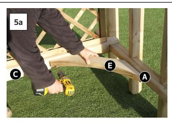
Ensuring Post C is perpendicular to Rail A, position Bracing E as shown in Fig.5 and fix using 2no 70mm Screws.
