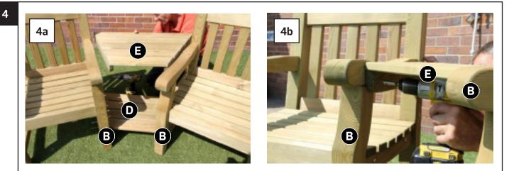
Position Upper Shelf Assembly E between seats and attach using 4no Screws - 2 per side (Figs.4a & 4b).
