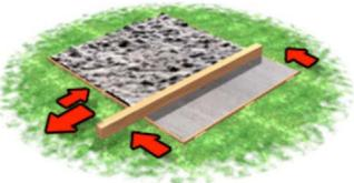
If wet weather is forecast, cover the concrete with polythene for 24-hours. In warm weather cover the base with damp sacks and sprinkle them with water over the 24-hour period, this will ensure the drying concrete will not shrink or crack.
