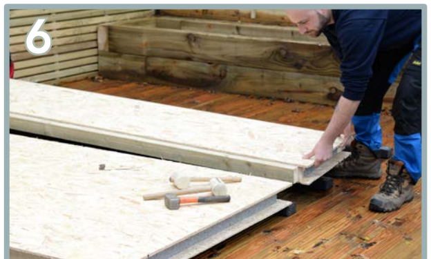
6 Place the second floor panel (E) onto the middle bearers. Ensure the panel is positioned half way on both bearers.
