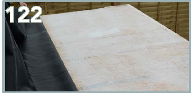
Apply glue to half of the roof and ensure to reach up to all of the edges.
