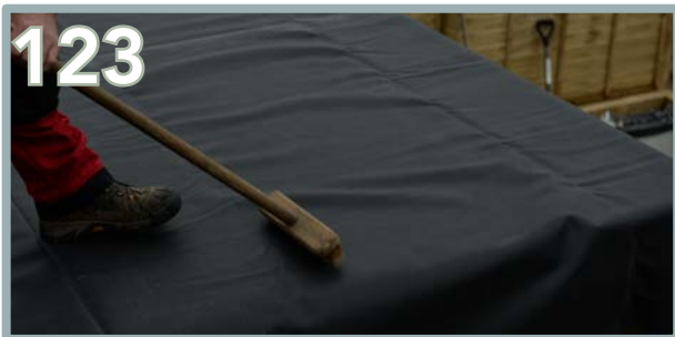
Roll the EPDM half way on to the glue. Use a brush/broom to create an even and flatter finish. You need to act quick once the glue has been applied.
