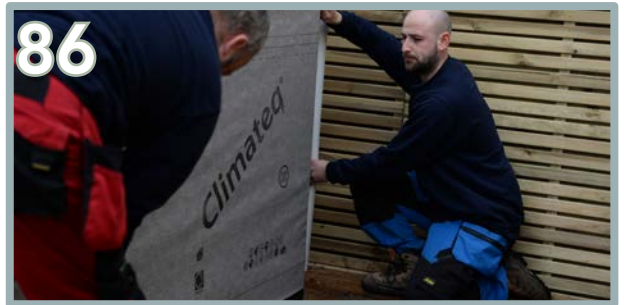
86 Continue unwrapping the membrane, pulling tightly and stapling into place.
