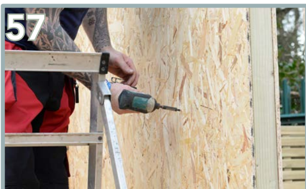
Internally position the screws each side of the adjoining split line. Use 5 x 35mm screws for each side of adjoining panels with the spline panel inside from top to bottom. Repeat this process for every adjoining panel.
