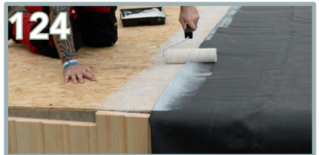
Repeat on the opposite half. Fold the EPDM back up until the point where the glue ended on the previous application.
