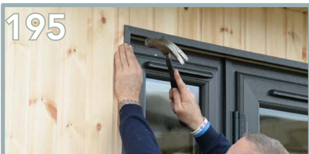
195 Use 5 x pins on the front down the side strip. Repeat the same process for the opposite side.
