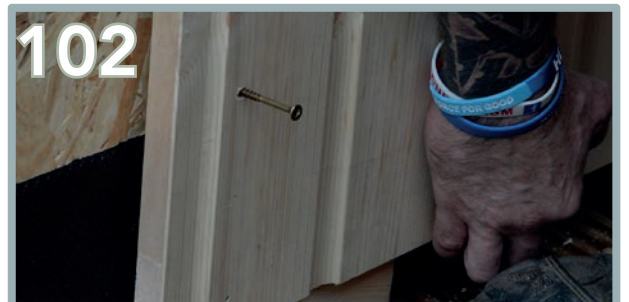
Use 6 x 80mm screws on each panel, 3 x 80mm down each side of the cladded panel, through the batten and into the wall panel behind. Leave the screws slightly out in case of adjustment.
