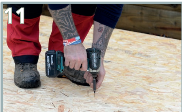
Once happy that all panels are in the correct positions, further secure with 5 x 125mm screws along the third panel edges and the first panels outer edge into the bearers beneath.
