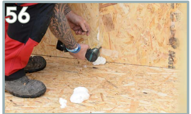
Repeat the process, using 3 x 35mm per panel internally.
