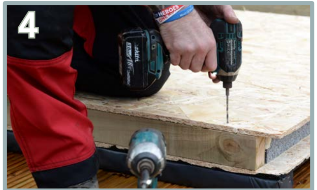
4 Pre-drill for every process before securing with screws. Pre-drill 5 holes along the edge of the first floor panel. Do not screw in the other side at the moment.
