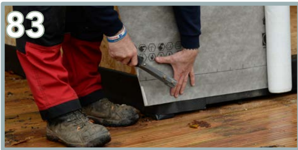
83 Begin to unwrap the breathable membrane. Position the membrane 45mm from the ground.
