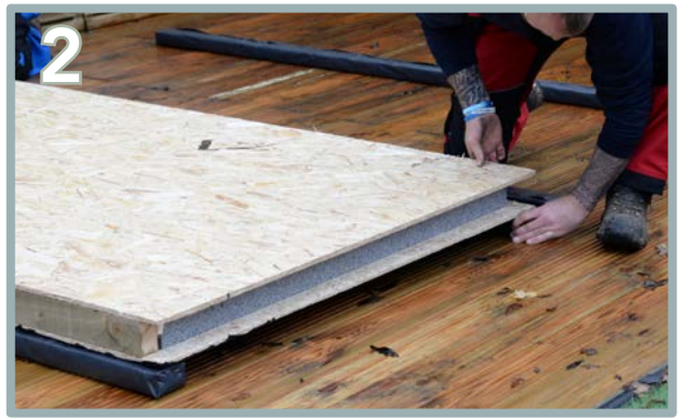
2 Place the first floor panel (D) on top of the two bearers and position it half way onto the second bearer. The black side covered in tar will be on top of the bearers as shown above.
