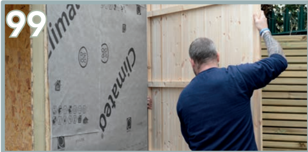
Begin applying the T&G cladding at the back (AZ).
