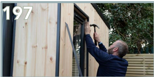
197 Pre-drill and use 5 x pins on the front of the side plastic trim. Repeat for the opposite side.
