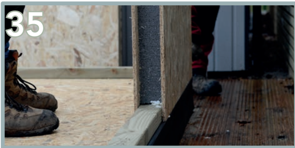
Place onto the floor plate and the wall panel will sit flush to the edge.
