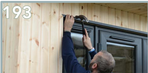
193 Pre-drill across the top and repeat the same process. Use 5 x pins across the front of the plastic trim.
