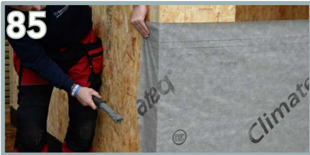
85 Then warp the excess around the corner and staple the starting point into place.
