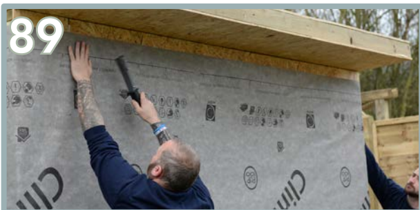
89 Add additional staples to keep the membrane in place. Be careful not to staple into the door and window gaps.
