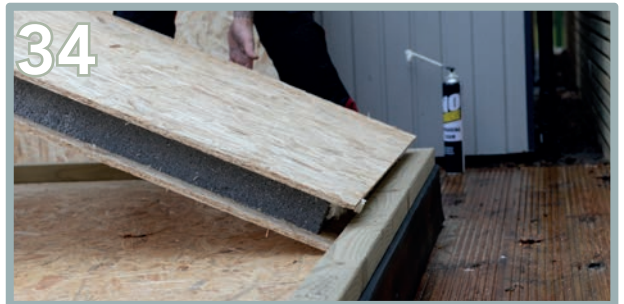
Begin the build at the left back corner, starting with Side Panel 4 (J). Insert the expanding foam provided into the bottom groove.
