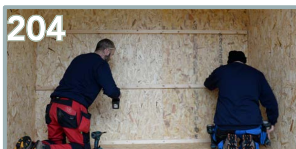
204 Using 5 x 80mm screws to secure in place.
