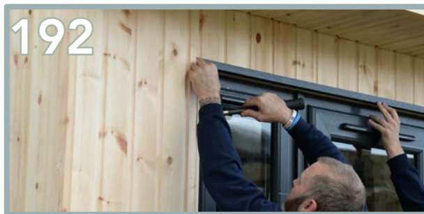
192 Using the pins provided with the trims, apply 2 in each corner and 1 x pin in the middle.
