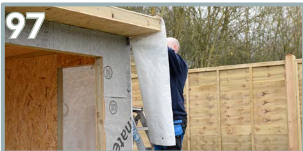
Remove the roof overhang excess.
