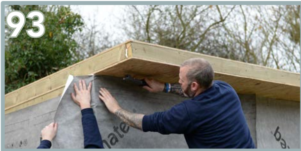
Using the excess membrane, cover the front flush up to the roof.
