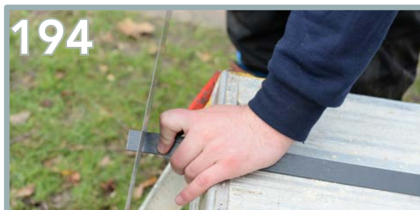
194 The side plastic trims for the door and window sizes will need to be trimmed down further to fit. Mark out your required length and cut.
