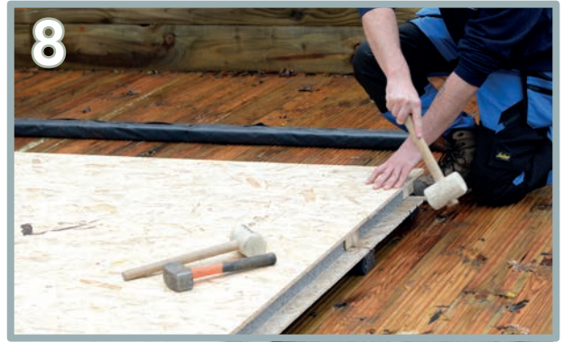
Knock on the front and back of the second panel to ensure it is flush on both edges to the first panel and floor bearers.
