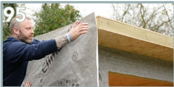
Use the excess membrane to cover the angle on the side panels.
