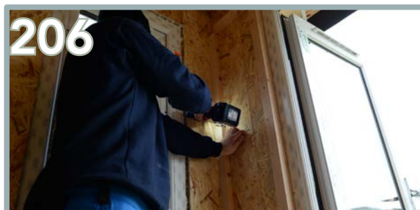
206 Using the 45x28x1960mm battens, apply one on each side of the door opening with 4 x 80mm screws. Then apply another two, with one in each corner, with 4 x 80mm screws.
