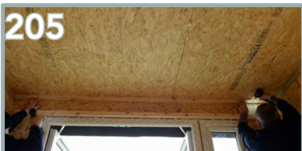
205 Apply one batten above the door opening, flush to the edge opening. Apply the top batten flush to the top. Use 5 x 80mm screws per batten.
