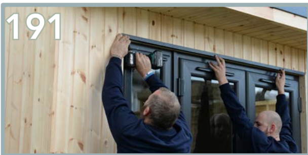
191 Position the top plastic 'L' strip across the door. Pre-drill the face underneath and fix first.
