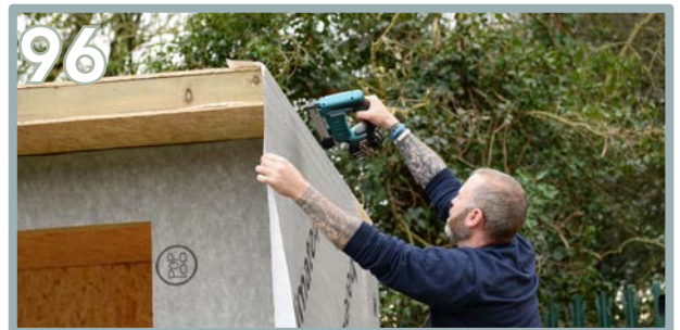
Fold onto the roof, stapling into place.
