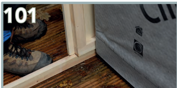
Repeat the same process for the second back panel (AX). Softly knock the second back panel into the first, so the T&G interlocks the panels together. Use a rubber mallet for a softer application.
