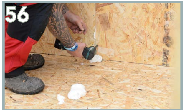
56 Repeat the process, using 3 x 35mm per panel internally.
