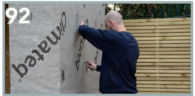
Repeat the same process to remove the excess from the window section.
