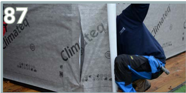
87 Once the starting point has been overlapped, cut off the excess and staple the end of the material into place.
