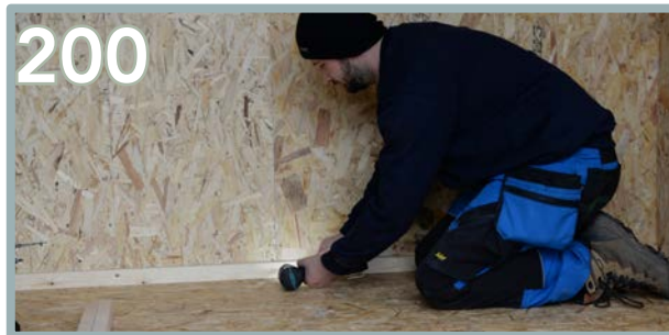
200 Repeat the process with the batten being flush to the bottom and end to end. Use 5 x 80mm screws along the batten at equal spaces.
