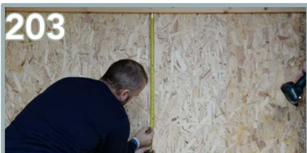
203 Repeat the same process to measure and mark out the position for the final back batten.
