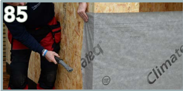
85 Then warp the excess around the corner and staple the starting point into place.
