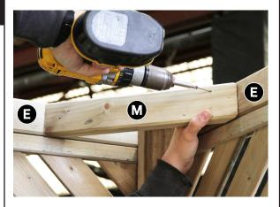
Attach Rear Corner Brace to Ring Beams E as shown in Fig.10 using 4x 60mm Screws –2x per side.
