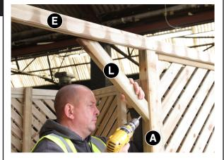
Attach Diagonal Front Brace L to Notched Post A and Ring Beam E using 2x 60mm Screws. Repeat procedure for remaining Diagonal Front Brace L.
