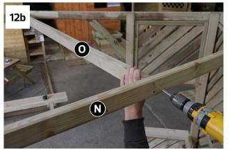
Locate Finial Support O between front Ring Beams corner and middle of Centre Brace N (Fig12a). Fix in position using 4x 60mm Screws as shown in Figs.12a and 12b.
