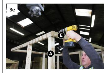
Locate Ring Beam E into notches of Notched Posts A (right side front facing the arbour), flush with Notched Post A as shown in Fig.3a. Using Side Panel J to set the distance between Notched Posts A, fix Ring Beam E in position using 4x 60mm Screws –2x per post.
