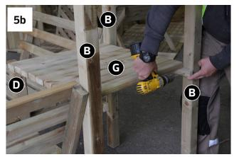
Position Table Top G onto Table Leg D and between Full Posts B as shown in Fig.5a. Ensuring Table TopG is levelled, fix in position through Table Top G battens using 4x 60mm Screws – 1x into each Full PostB & 1x into Table Leg D. See Fig.5b.
