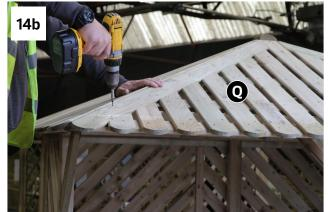
Position Roof Panel Q onto Finial P and Ring Beam E and attach to Finial P using 1x 60mm Screw as shown in Fig.14a. Repeat procedure for remaining Roof Panels Q. Ensuring Roof Panels Q are correctly aligned, fix to Ring Beams E using 12x 60mm Screws -3x per Roof panel Q -Fig.14b. Ensuring Roof Panels Q are correctly aligned, fix to Ring Beams E using 12x 60mm Screws – 3x per. Roof panel Q – Fig.14b.
