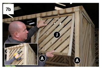
Locate 2x Side Panels J between Notched Posts A (ensure top Side Panel J meets underside of Ring Beam E and bottom Side Panel J is in line with the underside of Back Panel H) as shown in Fig.7a & 7b. Fix in position using 8x 60mm Screw -4x per Side Panel J. Repeat procedure for remaining Side Panels J.
