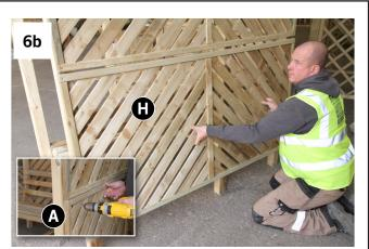
Attach 2x Back Panels H to posts to rear of seat assembly (ensure top Back Panel H meets the underside of Ring Beam E) as shown in Fig.6a and 6b using 12x 60mm screws –6x per panel. Repeat procedure for remaining Back Panels H.
