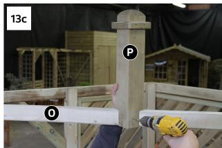
Locate Finial P onto Centre Brace N (1240mm from edge of front corner as shown in Figs.13a & 13b) and fix in position using 2x 60mm Screws –Fig.13c.
