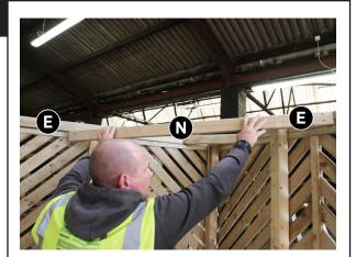
Attach Centre Brace N to Ring Beams E as shown in Fig.11 using 4x 60mm Screws -2x per side.
