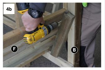
Position Back Rest F onto Seat C (Fig.4a) and fix in position using 4x 60mm Screws – 2x to Seat F (see arrows in Fig.4a) and 2x to posts (Fig.4b). Repeat procedure for remaining Back Rest F.
