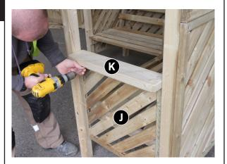
Attach Arm Rest K to Side Panel J as shown in Fig.8 using 2x 60mm Screws. Repeat procedure for remaining Arm Rest K.
