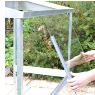
C. Fitting the glass
