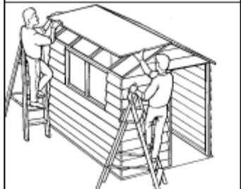
Now fit the roof. Using 60mm screws fix the roof from inside to either end. On the inside of your building there are roof spars that meet in the middle, fix these together using the triangle shaped roof ties using x4 40mm latt nails. This will help secure the roof and stop it from sagging.
