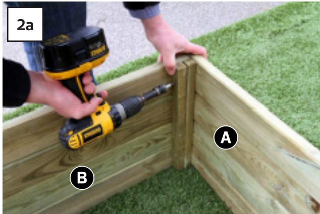
Secure in position using 8no Screws - 2no per internal corner (Fig.2a) and 12no screws - 3no per external corner (Fig.2b).
