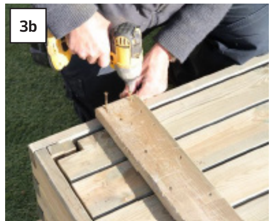
Invert the planter and place the base as shown in Fig.3a. Fix in position using 8no 70mm Screws – 2no per bearer (Fig.3b).
