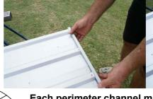
Each perimeter channel must finish flush with the edges of the sheets. the snap-tite system allows adjustment for this process by simply tapping the channel along the sheets until each end is neatly flush. If you need to remove channels from the panels, pull the channel along the panel from opposing ends. You may need someone to help with this.
